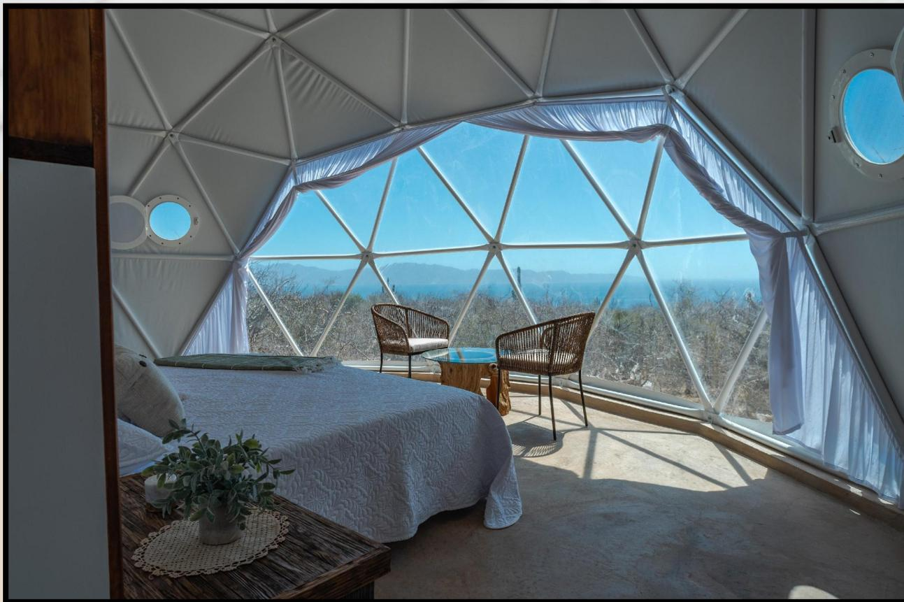
All of our structures are made with your choice of 1-inch steel or 1.5-inch galvanized steel struts. They are highly resistant to heavy winds, have a high snow load, and are protected against rust. Plus, we include a powder coat of electrostatic paint in the color of your choice to finish it off nicely and provide further protection against wear.
