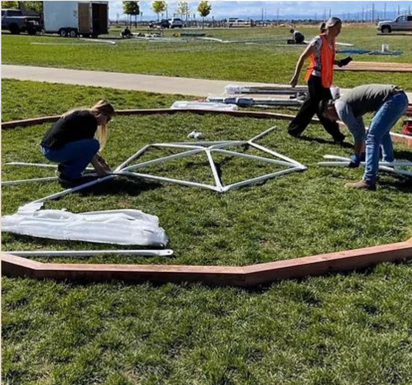
Creating a raised circular base for your dome is an essential part of your build. It will waterproof the interior flooring for your dome and also give you a secure place to anchor your cover. You have the option of buying the base from us (recommended) or we can give you the plans and specifications for you to make it yourself.
